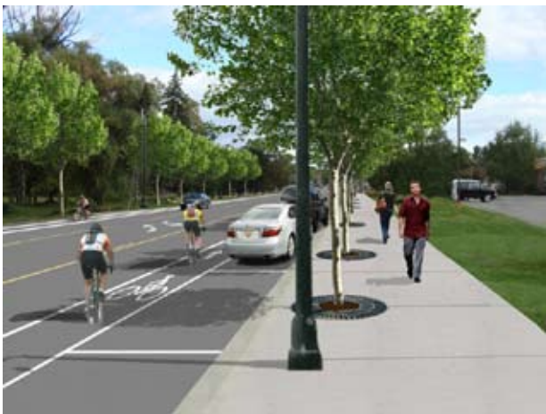
OPTION B – Reduction from 5 to 3 lanes with on-street parking, bike lanes, and sidewalks
